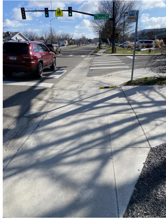
Figure 6: AB308 S Vista Ave & W Targee St NWC
